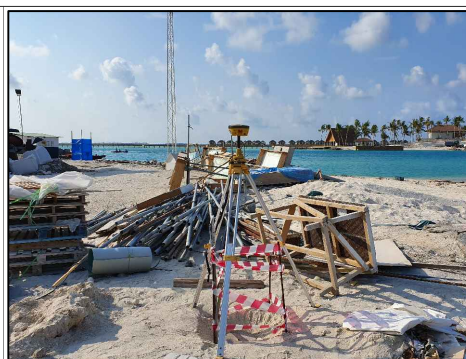
NORTH VIEW Distance 3m, height 1.2m
