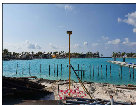
NORTH VIEW Distance 4m, height 1.5m
